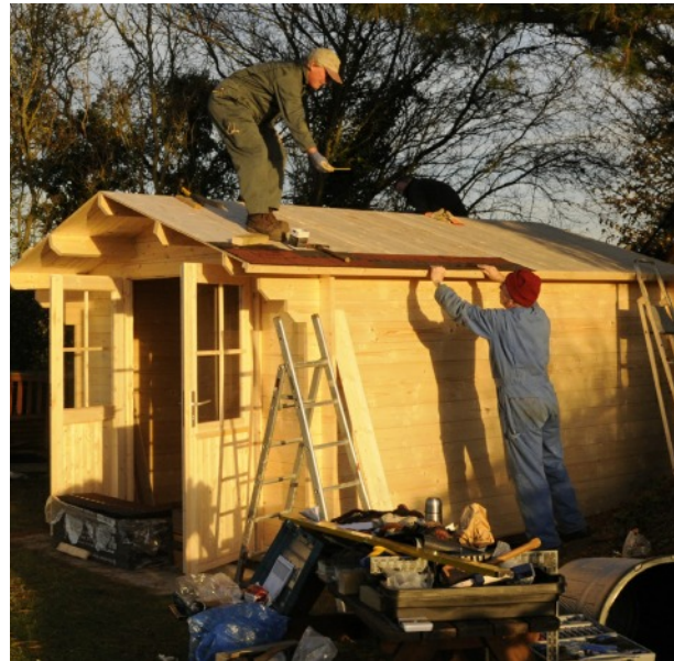
Andy, Malcolm & Chris busy constructing the new shed.
