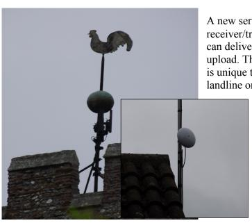
A new service is now available via a wireless receiver/transmitter installed on Bulmer Church Tower. It can deliver speeds of upto 32mbps for download **and** upload. The upload speed being equal to the download speed is unique to a wireless connection and not available via landline or fibre.
