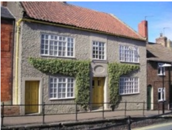
(Bethel Chapel on Cockpit Hill now used as a house)
