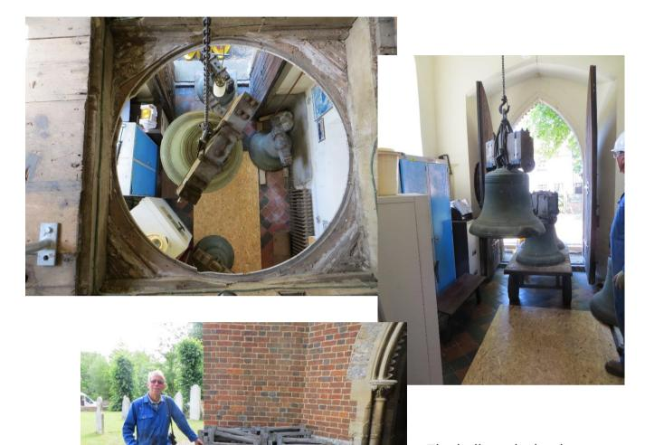
The bells and wheels finally removed and transported to the bell foundry at Loughborough for refurbishment
