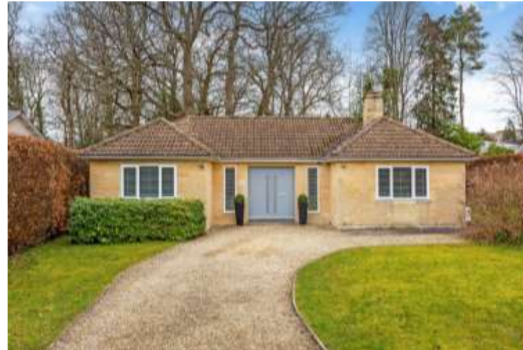
Building type: Bungalow
