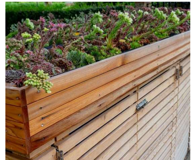
Hidden meters and refuse storage
