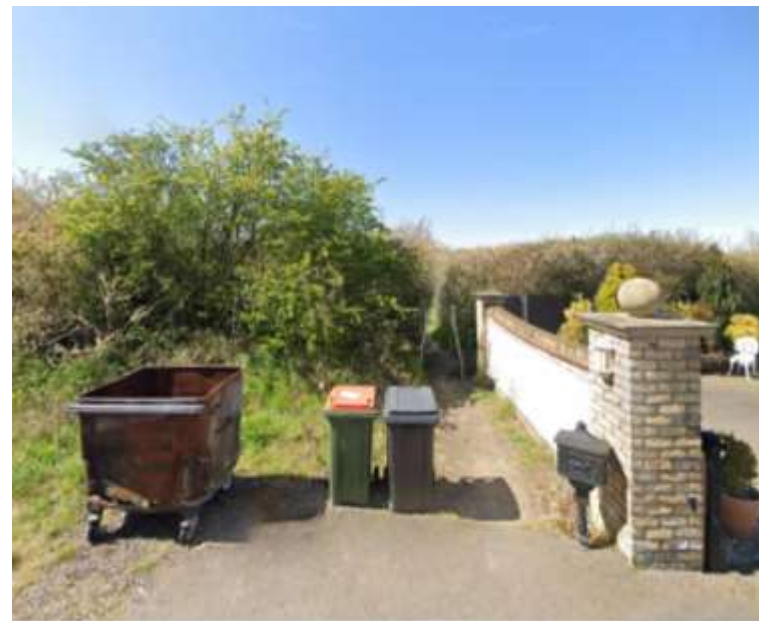
Poor access to public footpaths
