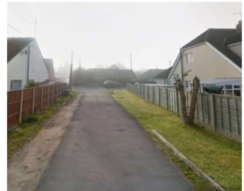
Poor oversight of the public realm.
