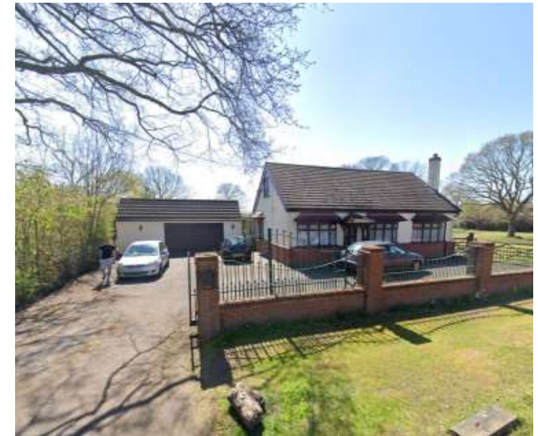
Garage roof complements the main building design
