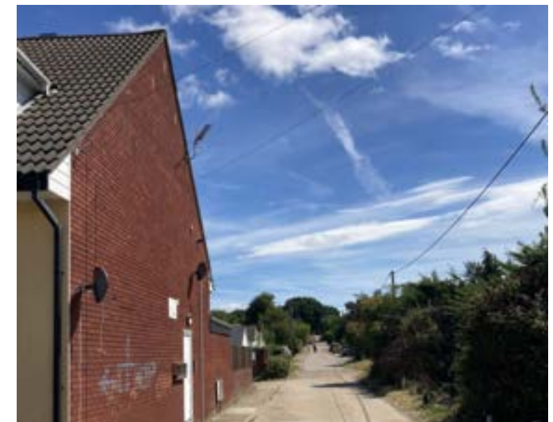
Blank elevations to public realm must be avoided
