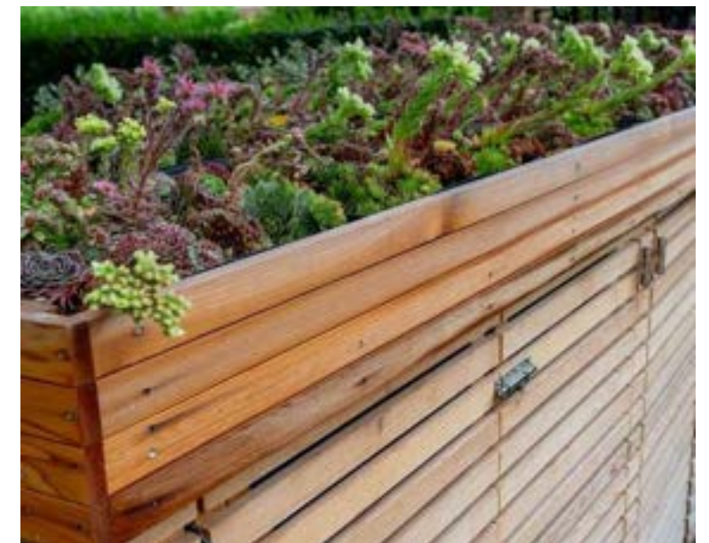
Hidden meters and refuse storage
