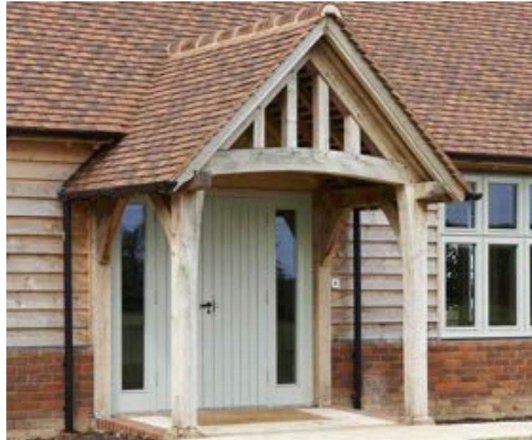
Porch design integrated into the building
