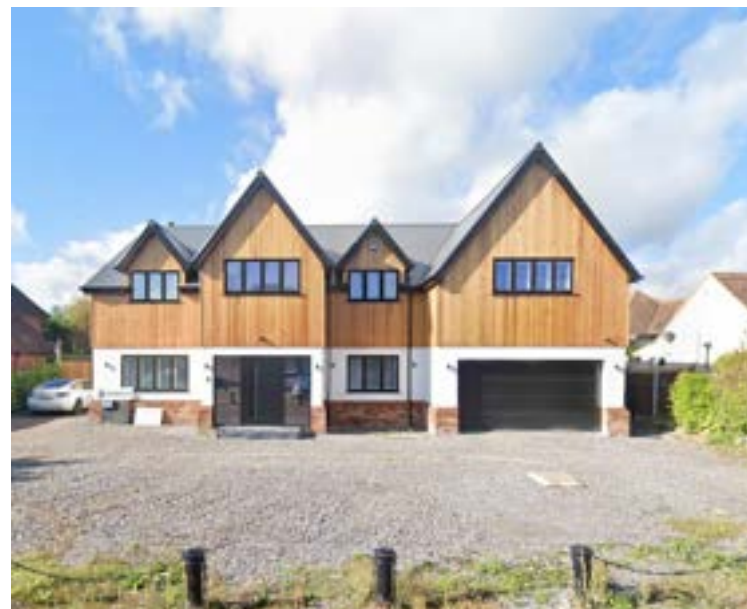
Garage forms part of the main building envelope
