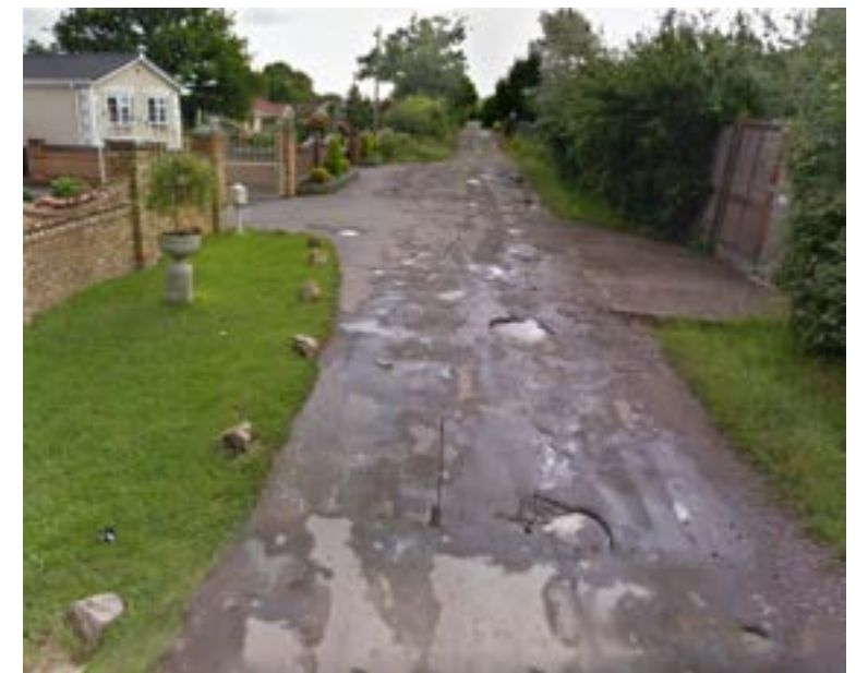
Existing Road: condition
