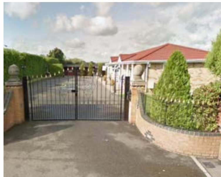
Building not orientated towards the street
