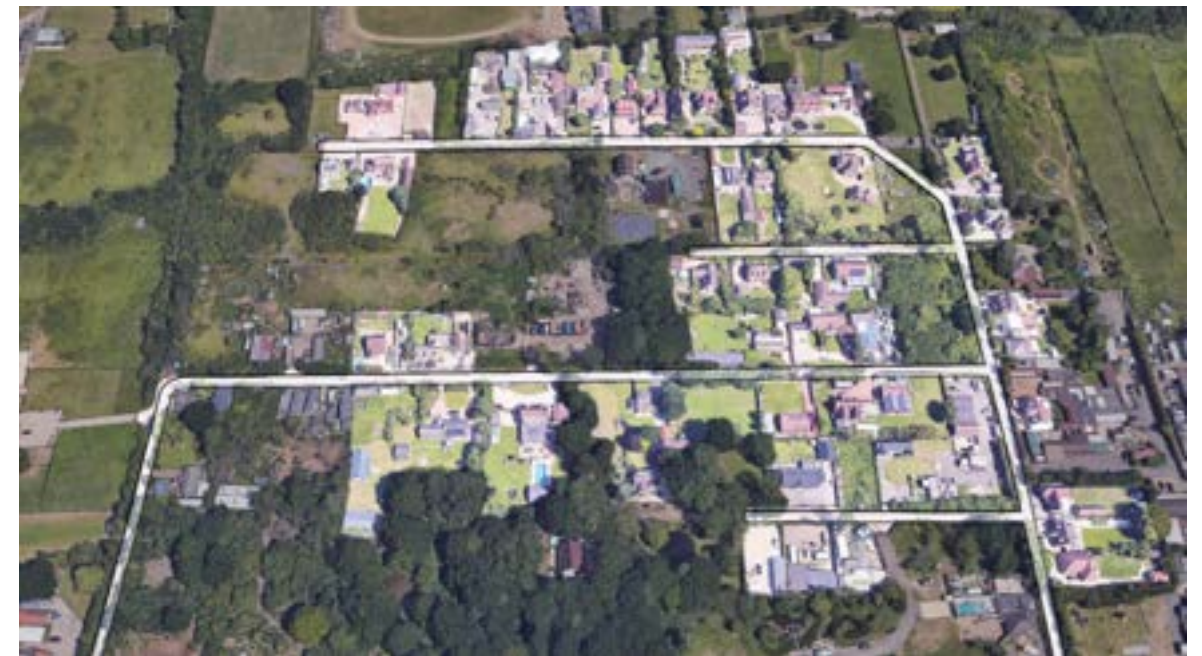
Unfinished block and incomplete road network
