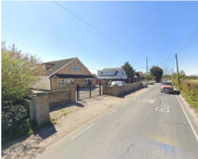
Existing dwellings along Burnt Mills Road
