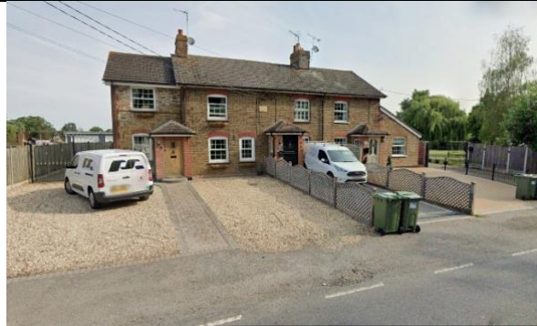
Wellington Cottage: South elevation from Burnt Mills Road
