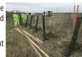
Image: Fencing works on A13/A130, January 2019
