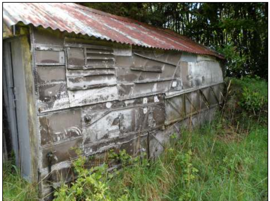
One of the sheds at Glomel with one wall made up entirely of Catalina components, at least some of which are from the internal wing structure Charles Street
