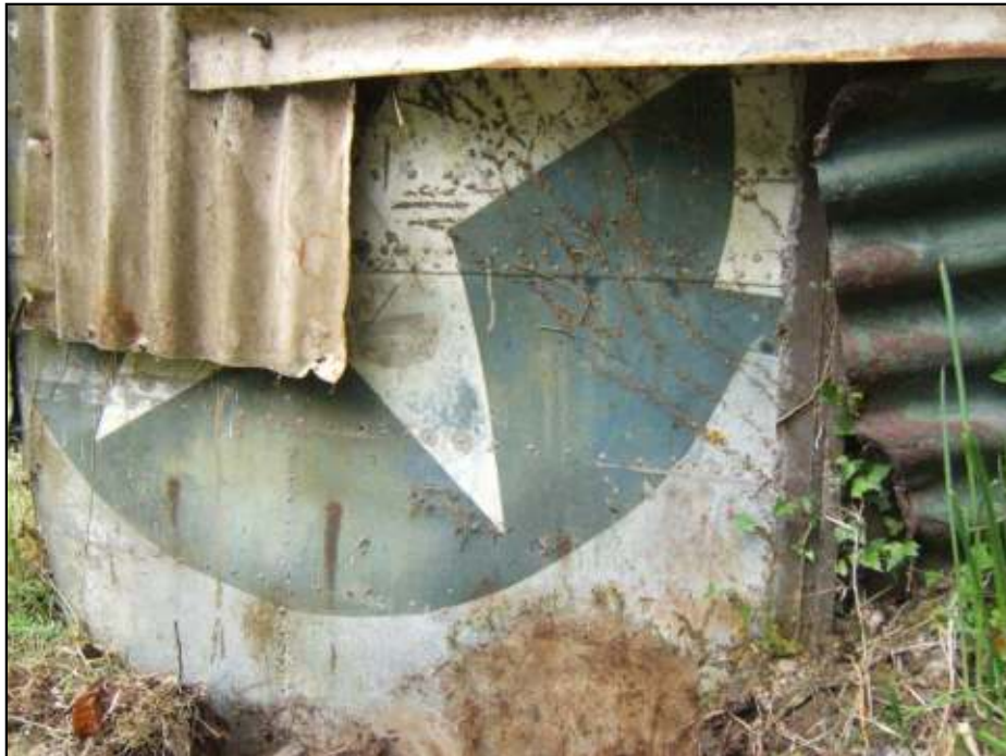
One of the sheds at Glomel in France partly made from Catalina components. The US 'star and bar' insignia looks as if it was originally from the forward section of the hull Charles Street
