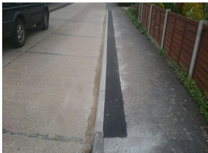
Chestnut Road Highways Devolution Works - After
